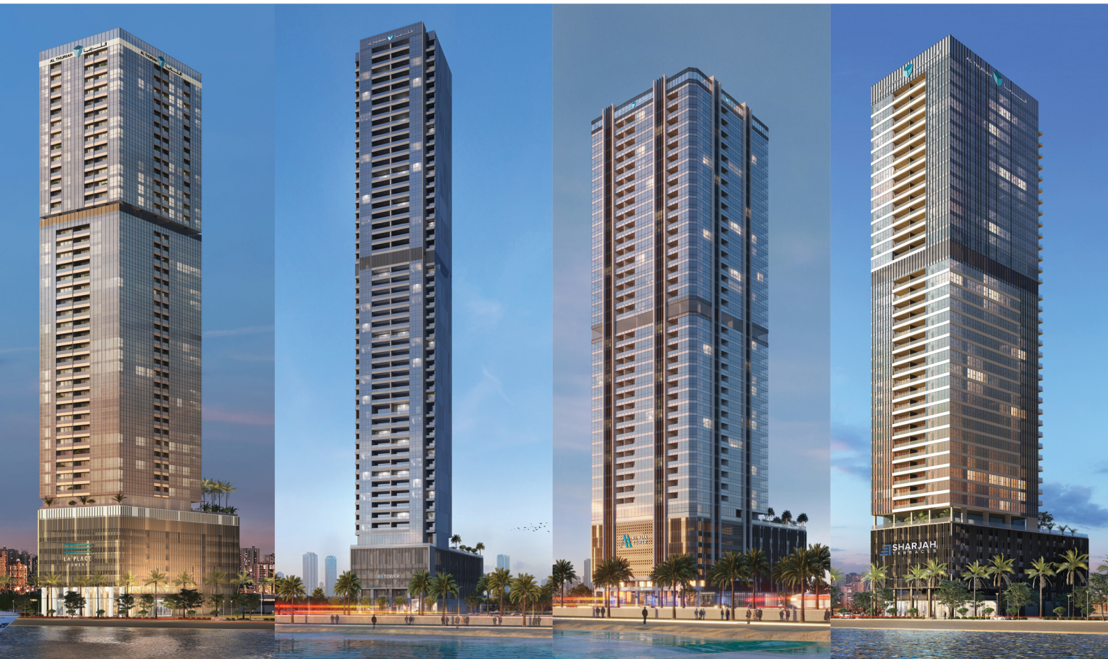
From left to right: La Plage Tower 2, 88 Tower, Al Alia Tower and Sharjah Terraces
