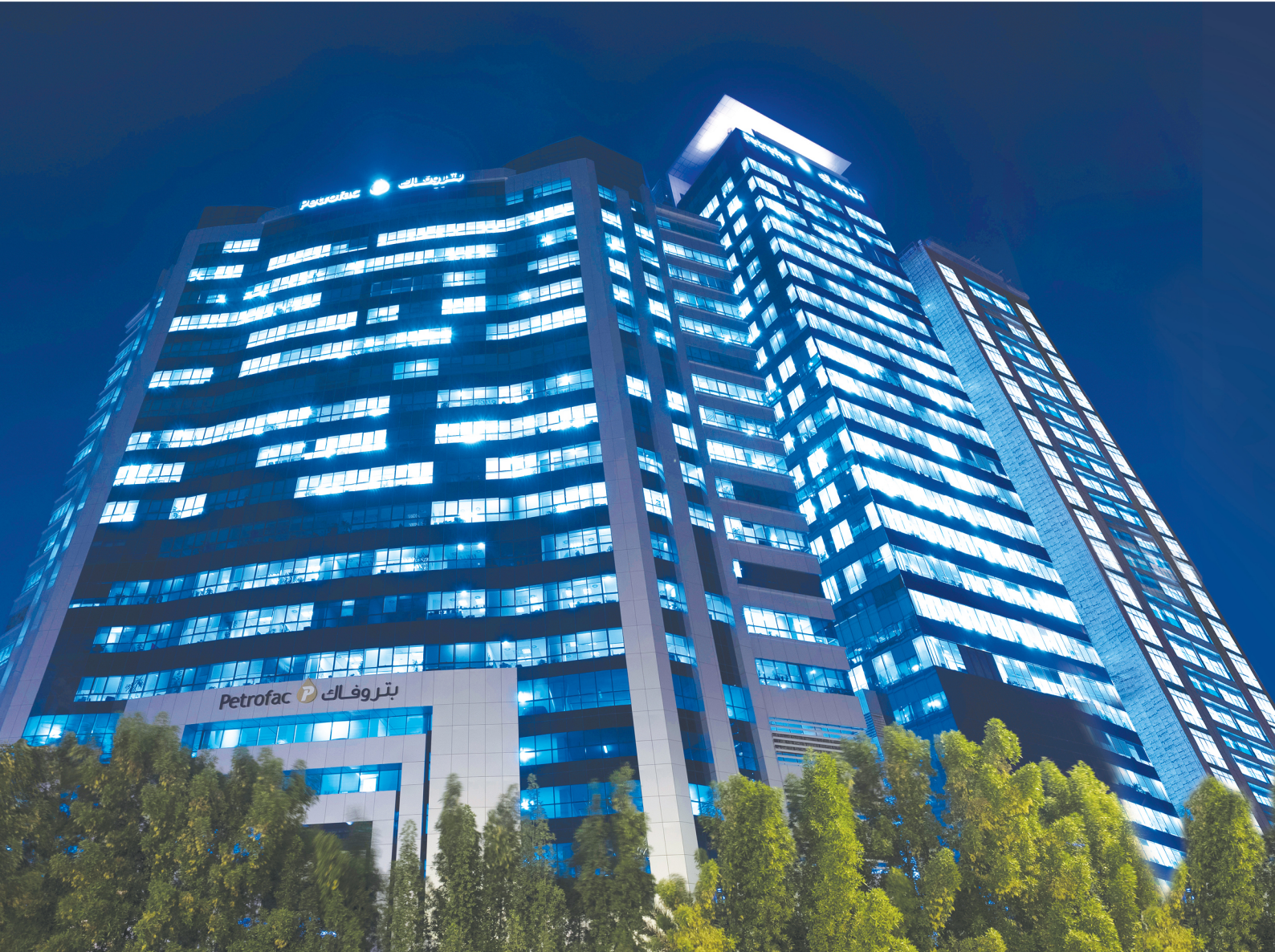
Petrofac Tower 1 and 2, Al Khan, Sharjah
