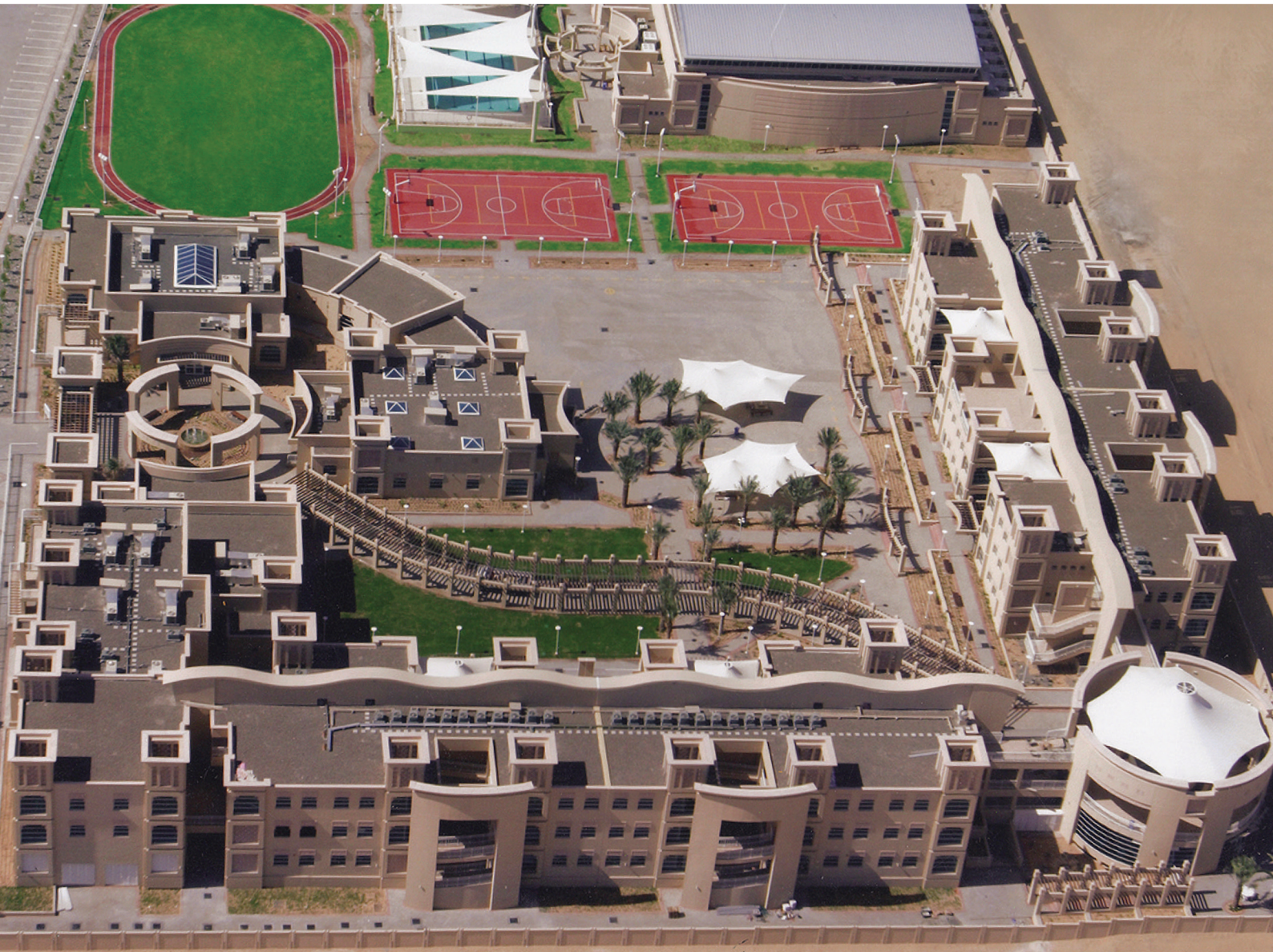
Lycée Georges Pompidou, Al Ruwaya, Dubai
